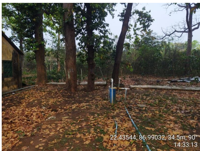
Lifting of water( HP pump)
